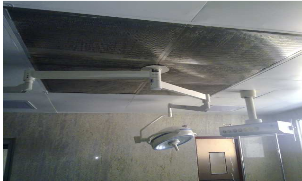
Picture - 1. Air -Filters - Operation theatres
